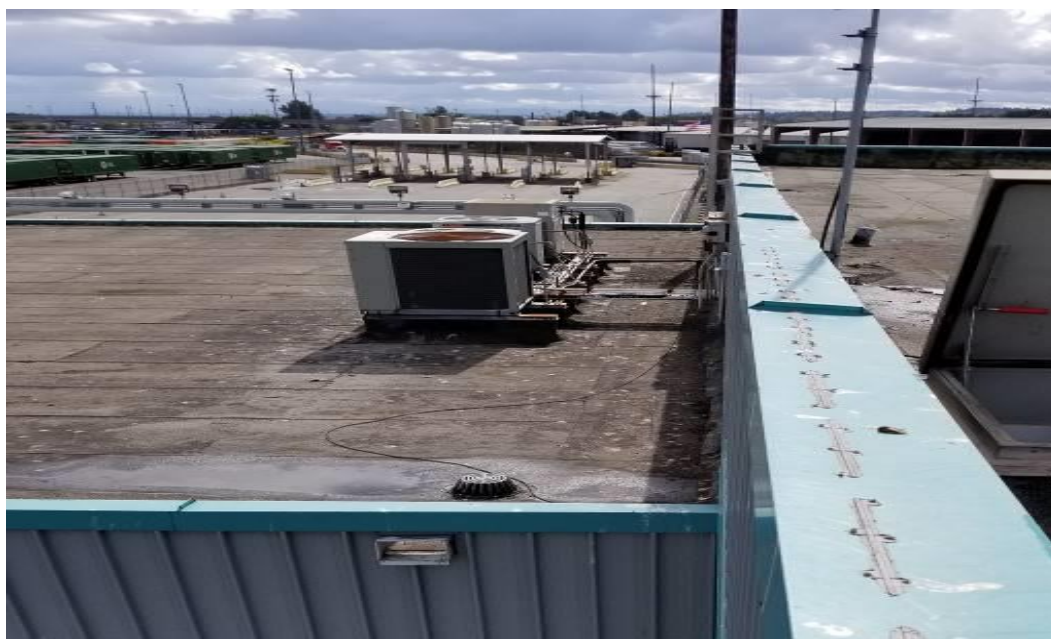
Photograph 4: Lower roof, HVAC system with no fiberglass insulation on ducts.
