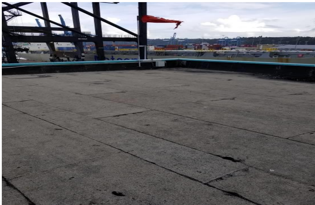
Photograph 2: Built-up roof system, Upper roof.
