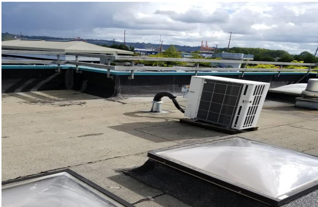
Photograph 3: Built-up roof system, Middle roof.
