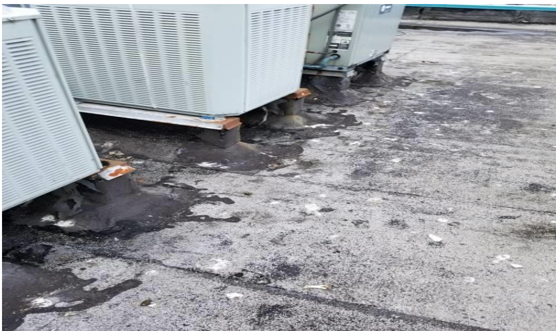
Photograph 5: Lower roof, HVAC system, sample 20 location, black sealant at the base of HVAC units.
