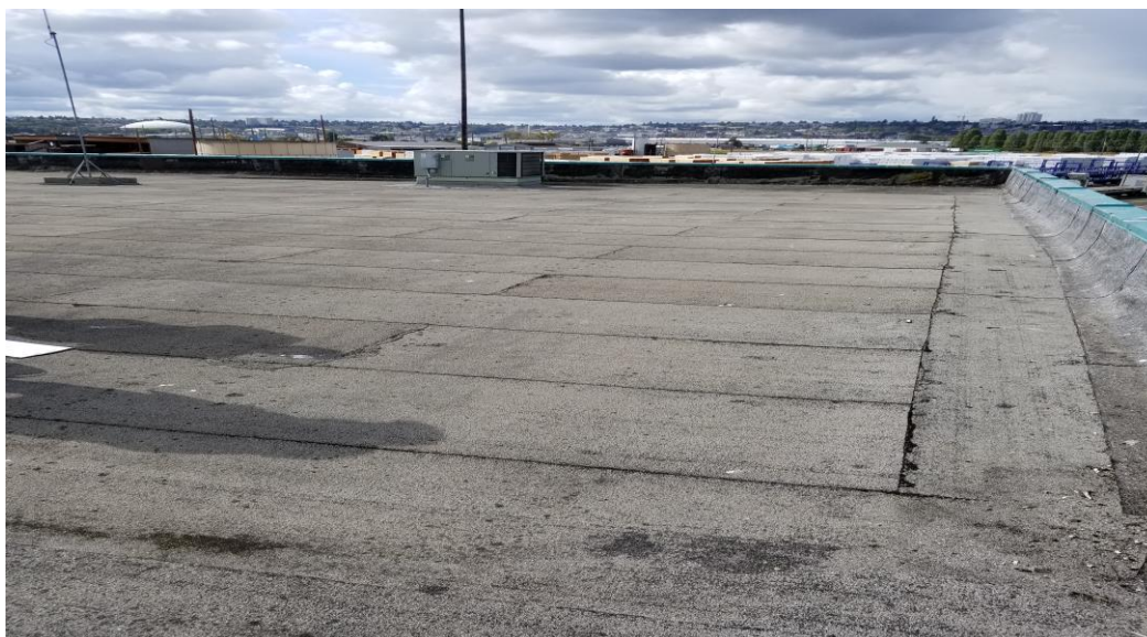
Photograph 3: Upper roof, Built-up roof system and HVAC system with no fiberglass insulation on ducts.
